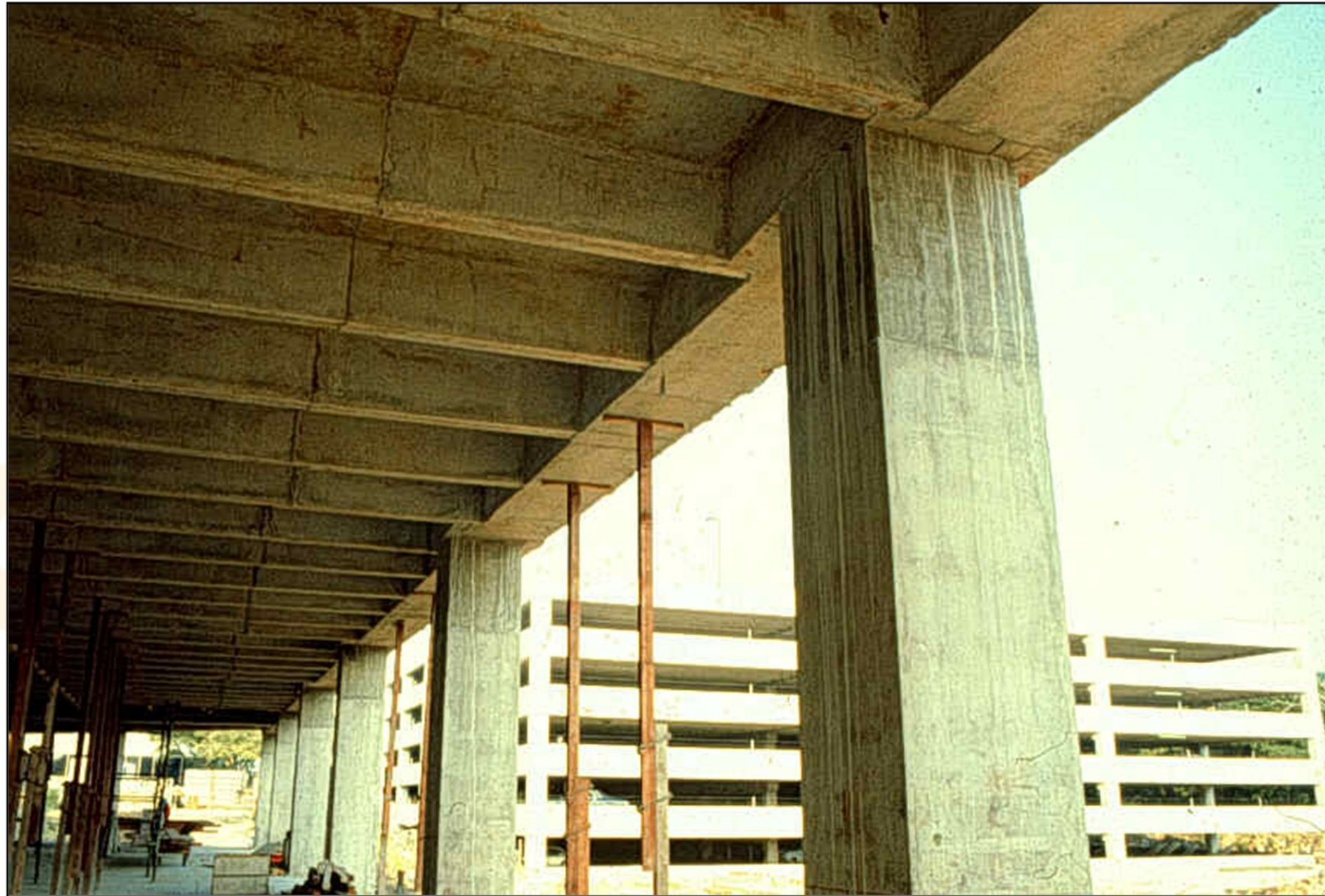
View of Pan Joist Slab from Below
