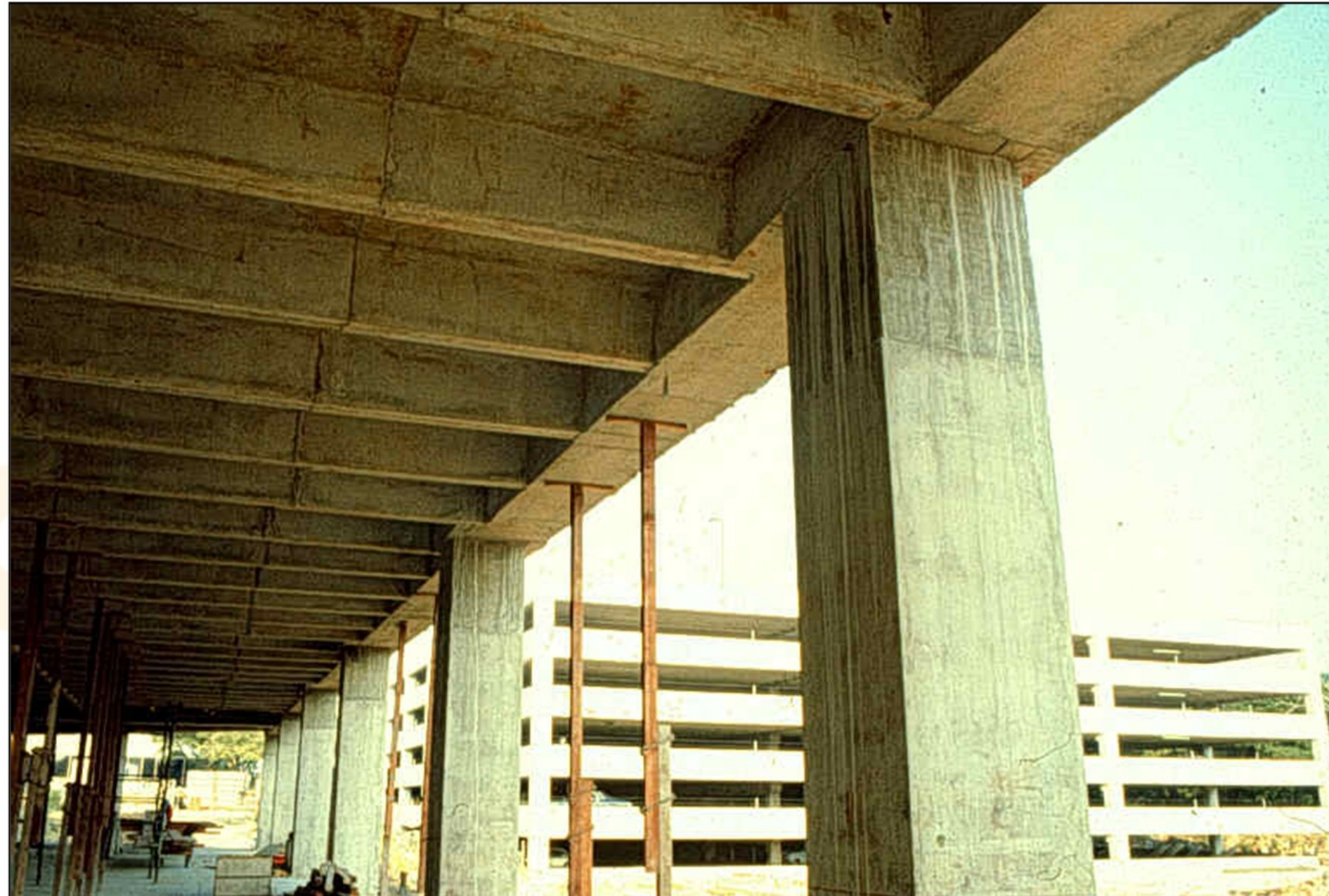
View of Pan Joist Slab from Below
