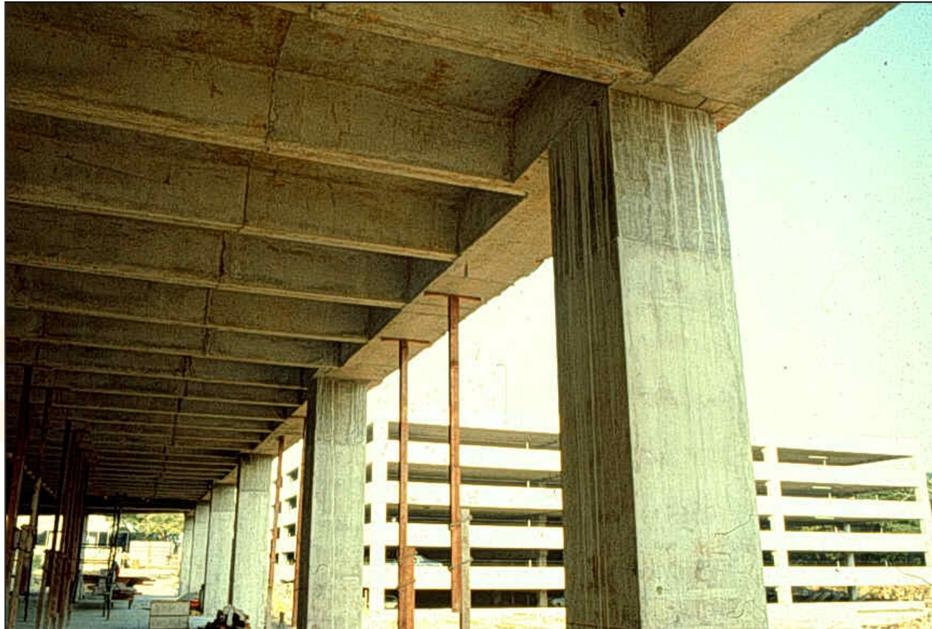
View of Pan Joist Slab from Below
