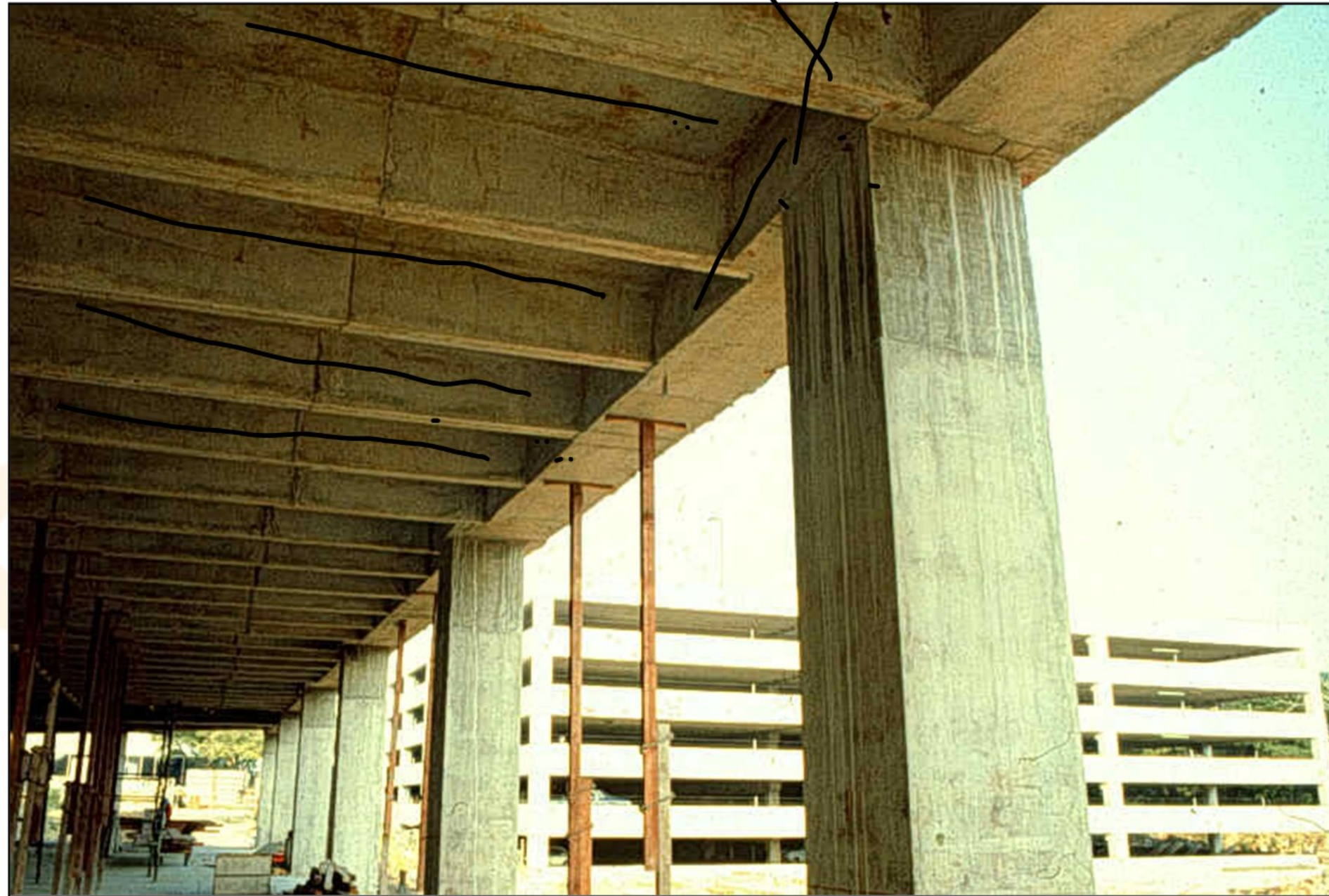
View of Pan Joist Slab from Below
