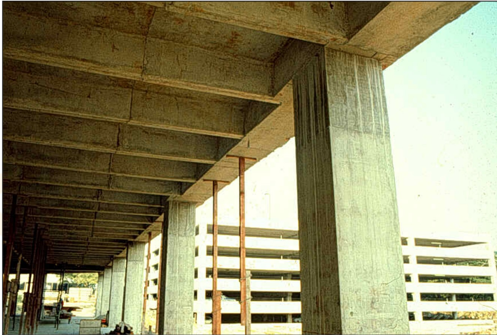
View of Pan Joist Slab from Below
